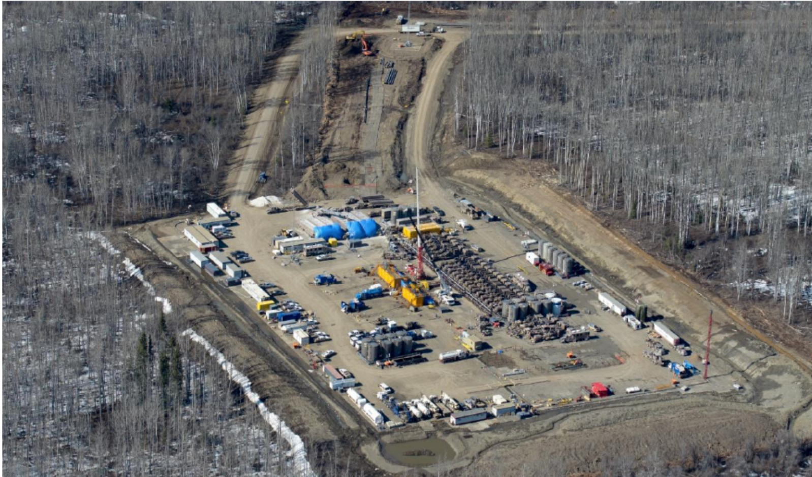
Figure 13. The Apache 34 pad in the Horn River Development of Northern British Columbia is a total of 6.3 acres where twelve multiple fractured horizontal wells recover gas from approximately 5000 acres.
