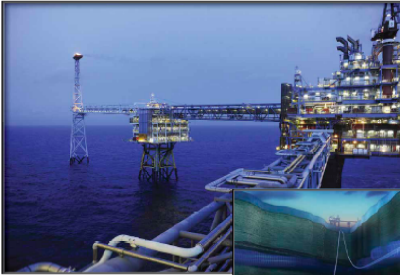
Liquid carbon dioxide has been injected into the Sleipner gas- and oilfield in the North Sea for 15 years without triggering any seismicity. It serves as a good example of how fluid injection can be done safely.
